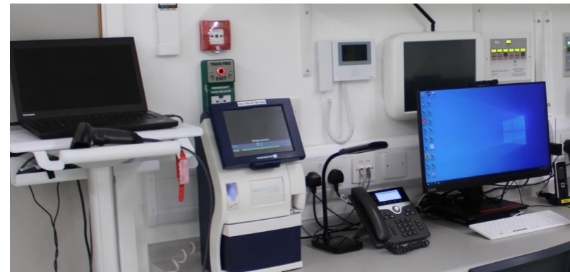
Digital equipment. Source: WUTH Library
